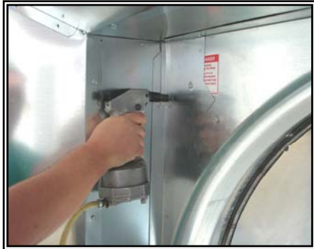
Figure 5 – Fasten with Pop-Rivets
