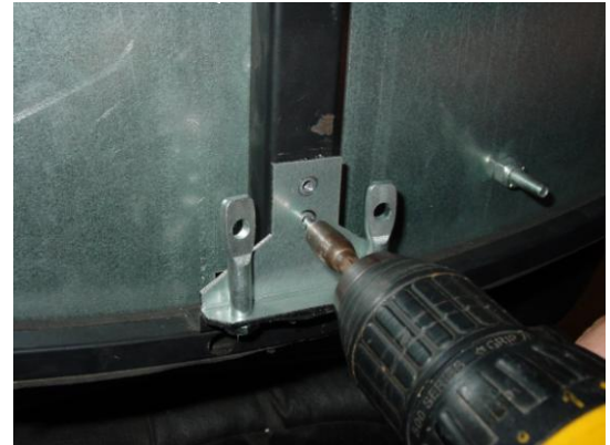
Figure 3 Drill Tek Screws
